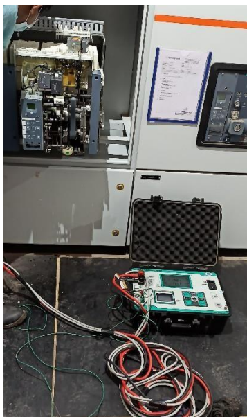
Air circuit Breaker Testing
